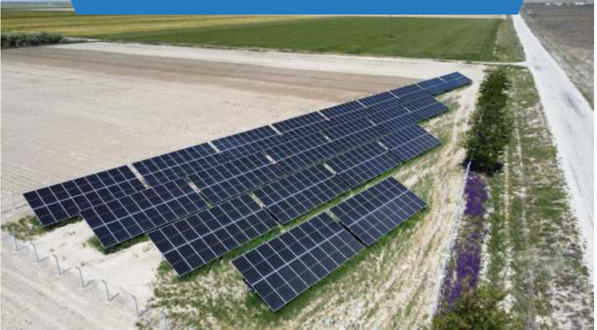
Ramazan Akdoğan | 210 kWp | KARAMAN - Burunoba
