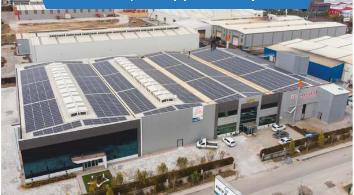
Mvs Volan | 721 kWp | KONYA- Selçuklu
