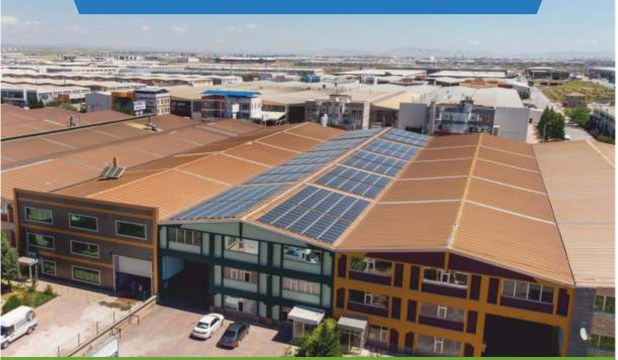
Apsan | 1200 kWp | KONYA - Karatay
